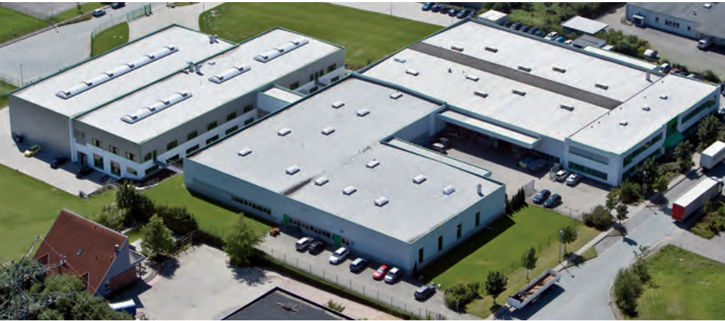
Headquarter in Bad Oldesloe – on 9200 m 2 production and office area nearly 400,000 valves are produced every year
