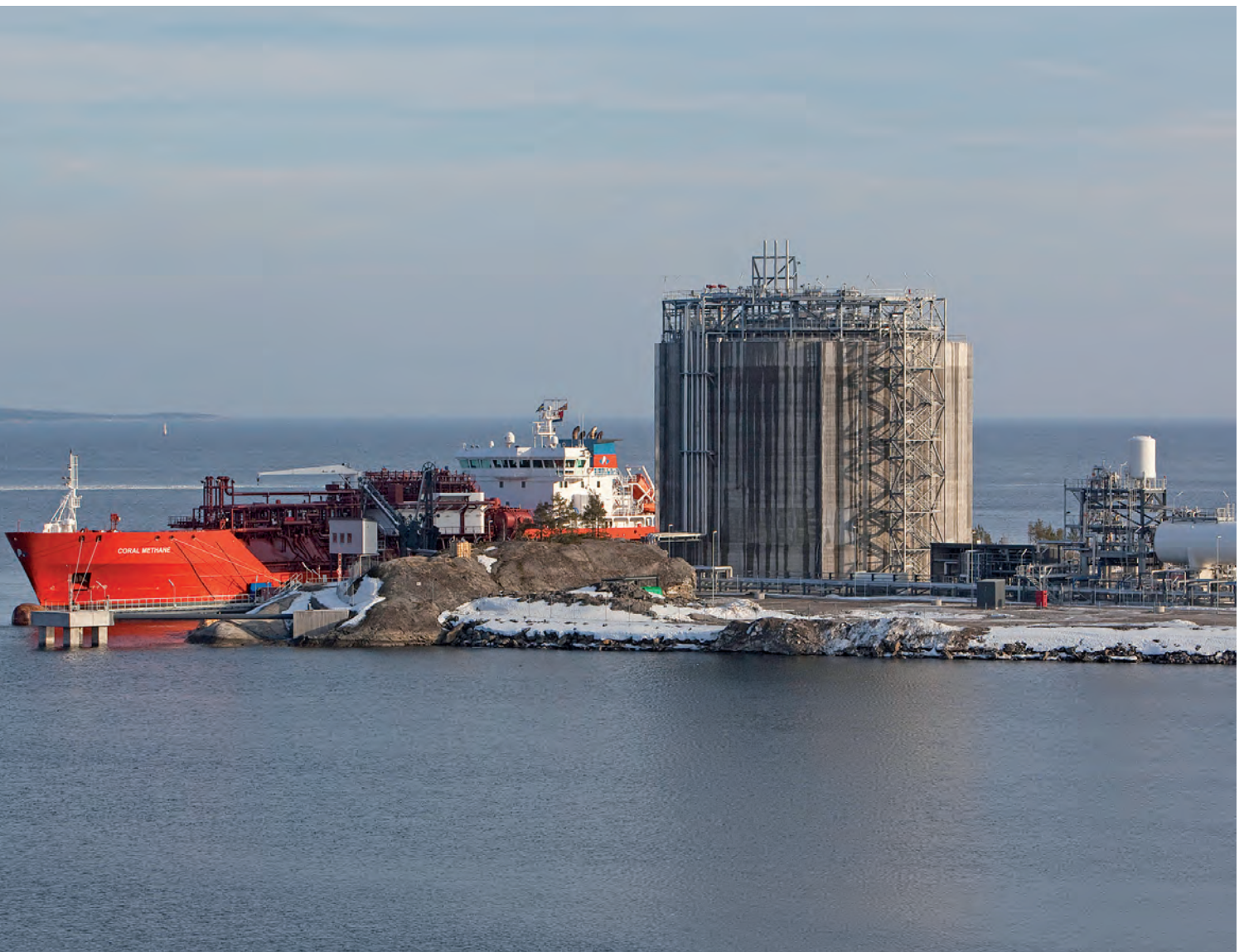
The LNG Terminal in Nynäshamn, Sweden. Equipped with HEROSE Valves for cryogenic applications
